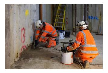
TamPur 130 / TamKat 130 is a single-shot hydrophobic polyurethane based on MDI in combination with polyether polyols and an amine based catalyst. The system only reacts when it comes into contact with water, producing a semi-flexible polyurethane foam.
